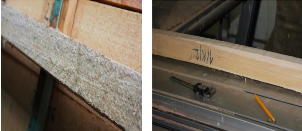
Fig. 1 Initial longitudinal warping and the woolly appearance surface of tested timbers.
