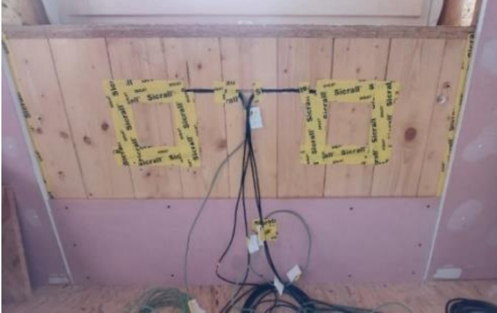
Fig. 5 Installed sensors in the construction of MHM exterior panel wall.
