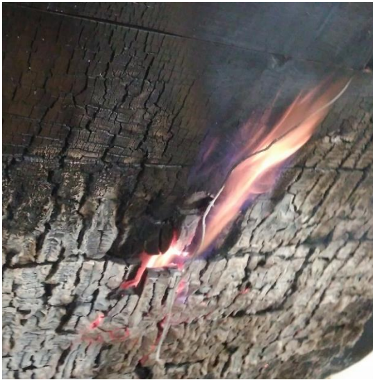
Fig. 2 Char layer fall-off during the medium-scale test.
