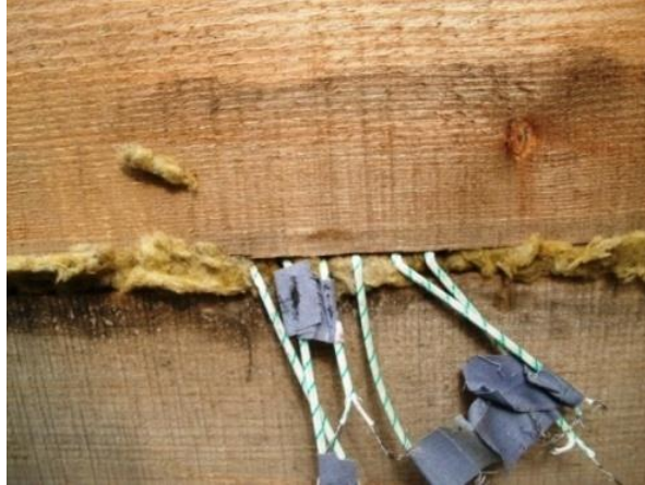
Fig. 11 Unexposed side of their test sample with the mineral wool insulation after thermal loading for 60 min.
