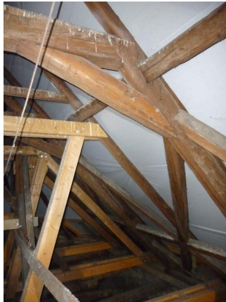
Fig. 5 Truss above the southern chapel, Liegender Stuhl
