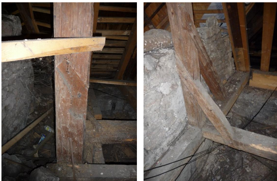
Fig. 6 Different details of upward braces
