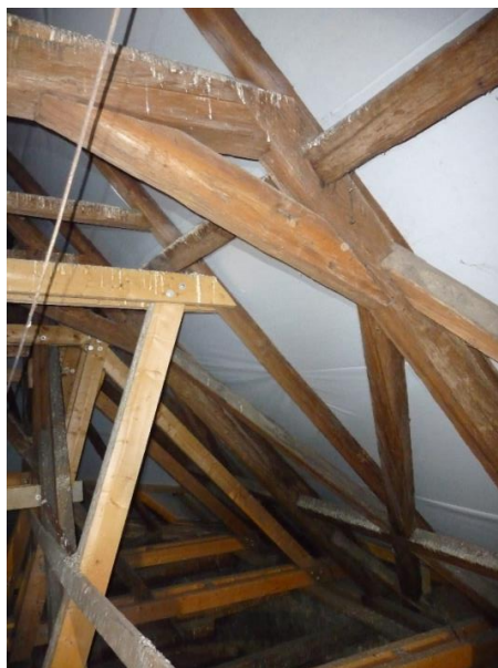
Fig. 5 Truss above the southern chapel, Liegender Stuhl
