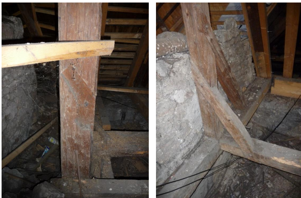
Fig. 6 Different details of upward braces
